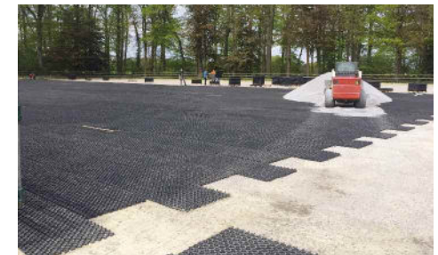
Mats are laid over a drainage layer
